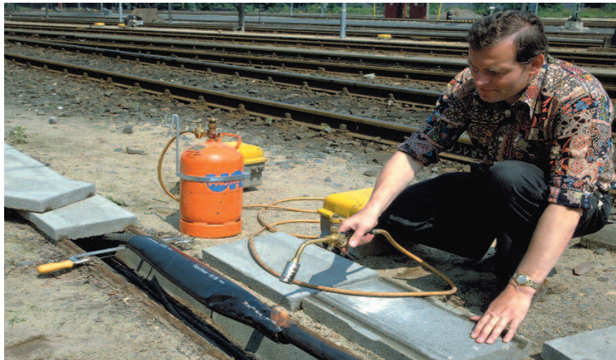
Picture : The Armarap joint case allows the electrical and mechanical functions of the cable armour to be restored simply and quickly.
