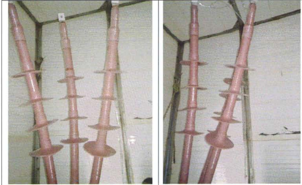
Photographs showing the sample Outdoor terminations Before 1000 hours Salt-Fog test.
